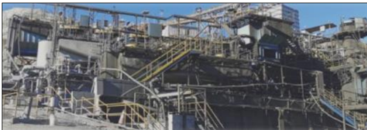
Figure 5-11: Process Plant Overview – Flotation Circuit in Foreground
