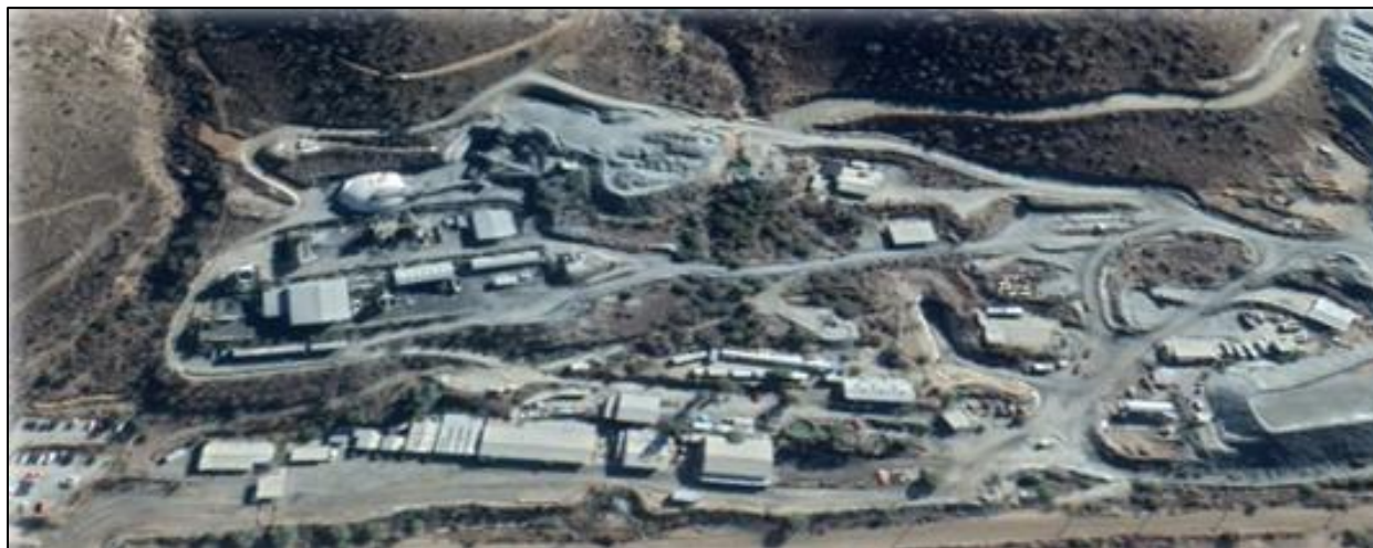
Figure 5-10: Los Mantos Process Plant Overview
