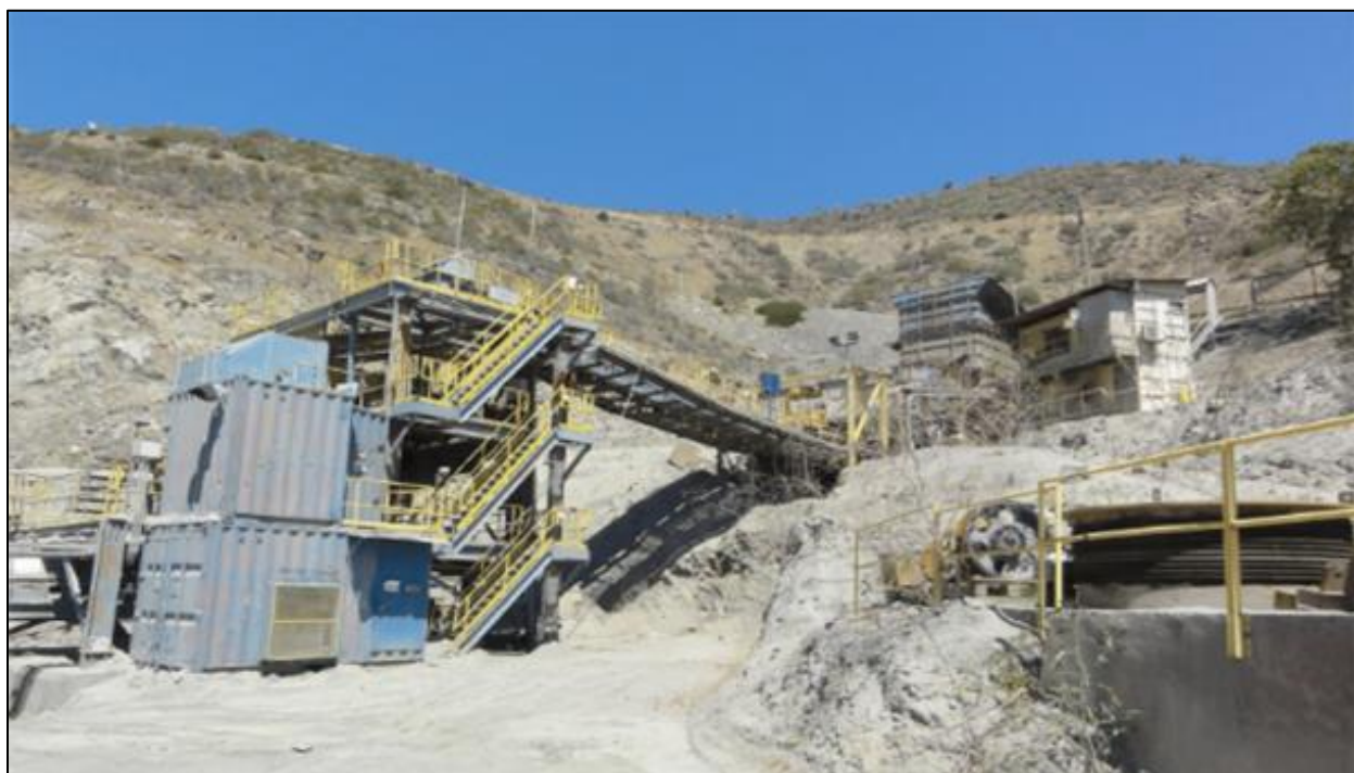
Figure 5-12: Process Plant – Crushing Circuit
