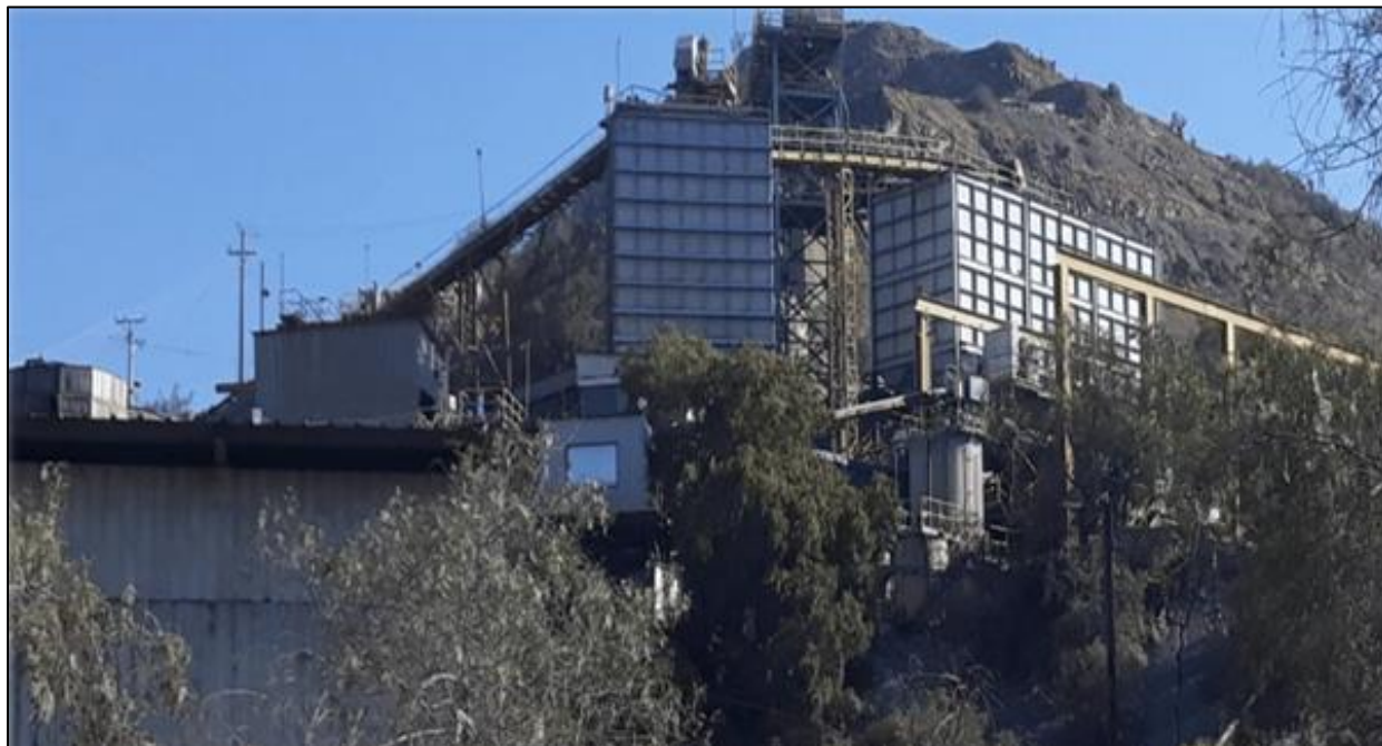
Figure 5-13: Process Plant - Grinding Circuit
